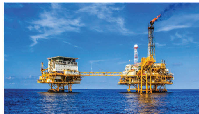
Gas leak detection
